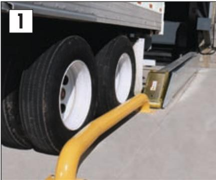
1 As the vehicle approaches the loading dock, it is guided into position between the wheel guides.
