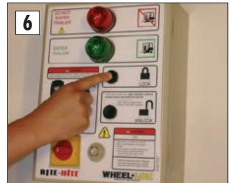
6 the dock attendant inside pushes the "lock" button on the control panel to activate the locking assembly.
